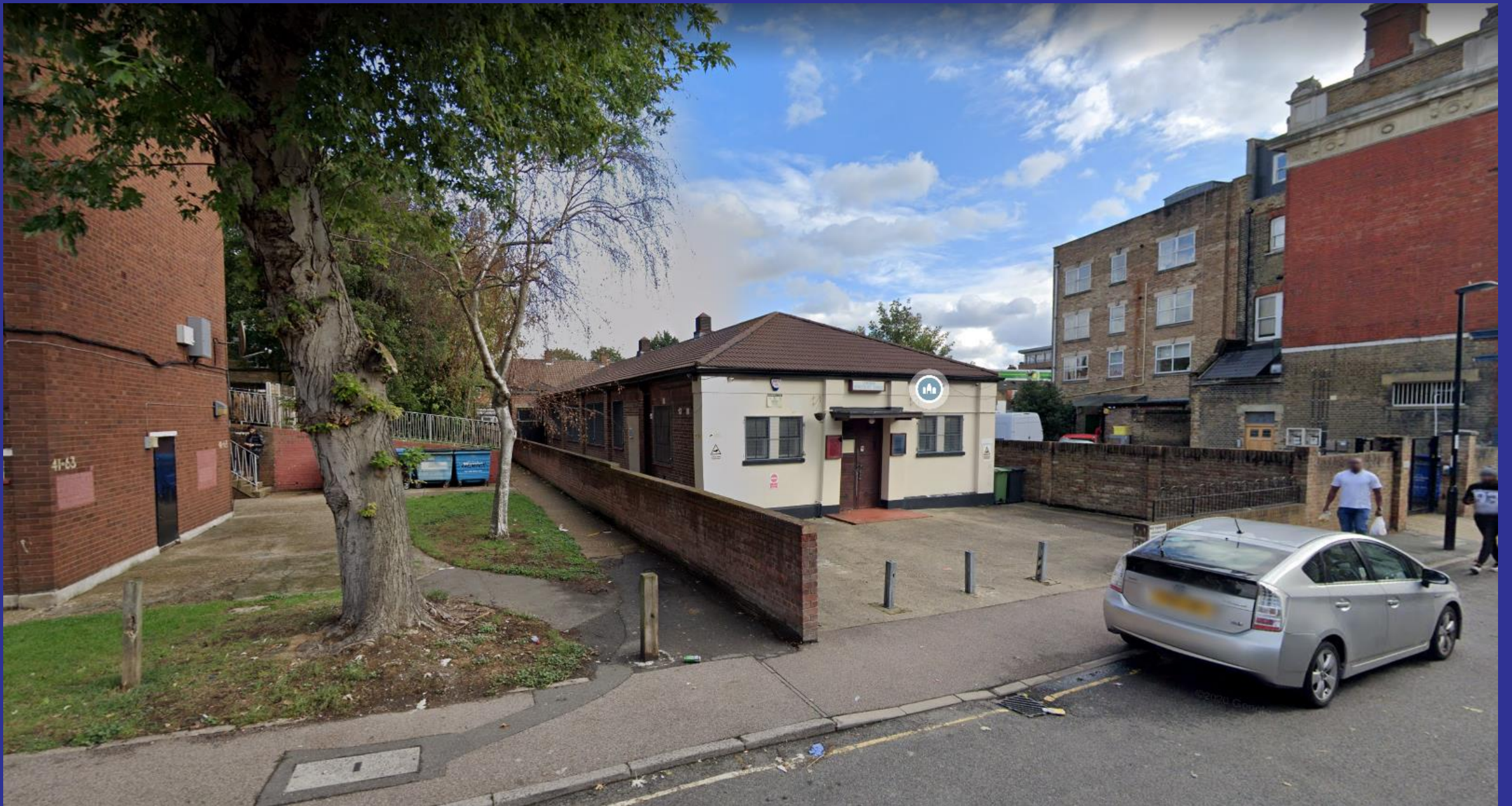
Front Elevation Photograph
